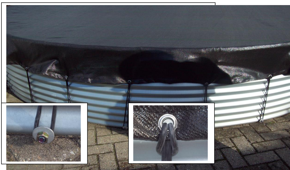
Fig 1: Anti-algae tension sheet installed on silo
